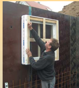
Nail up the inside wooden support
