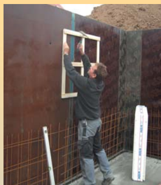
Nail up the wooden support frame
