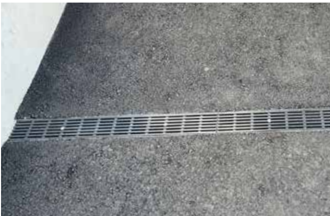
Driveway: 100V line with longitudinal GRP bar grating, charcoal grey
