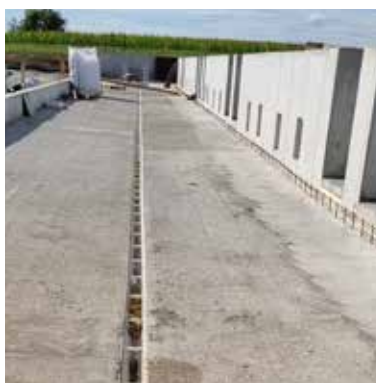
Slotted GRP design grating, charcoal grey
