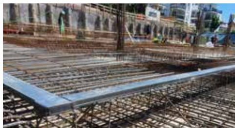
Installation AquaStop with gutter elevation
