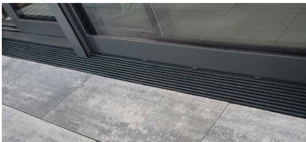
In the picture, the gutter was placed on drainage mortar and drilled open
