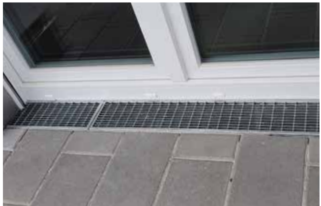
Patios: Fixo 150 with pressure-locked grating 30/10
