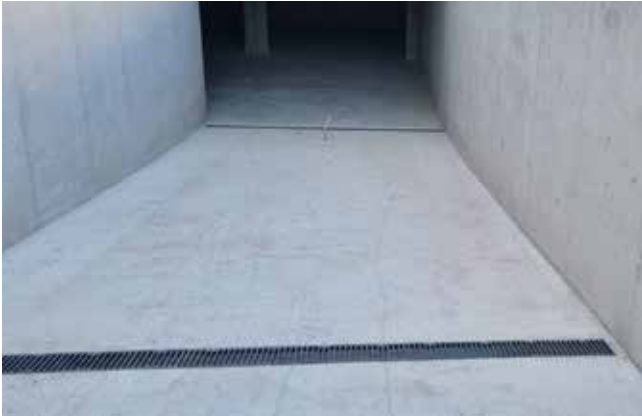
Entrance/exit ramps 150V line with cast iron grating
